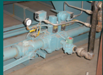
SCC Integrated Gas Valve/Actuators/Regulators
